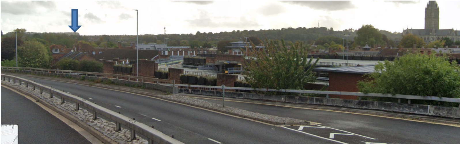
View of site from Ring Road
